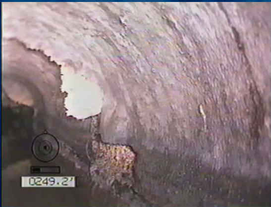
Negative side water pressure
