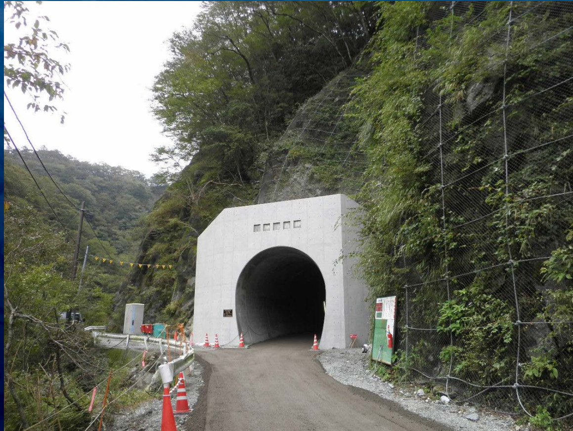
The local tunnel of Kanagawa Prefecture (L=275.2m)
