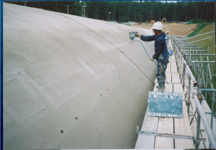
Xypex spraying
