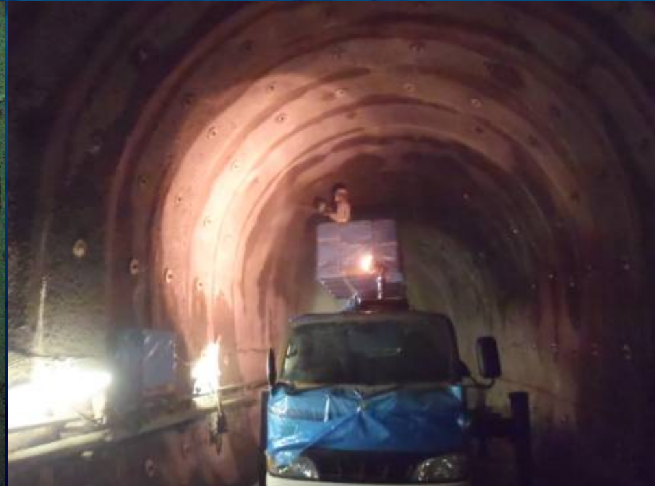
Xypex Spraying
