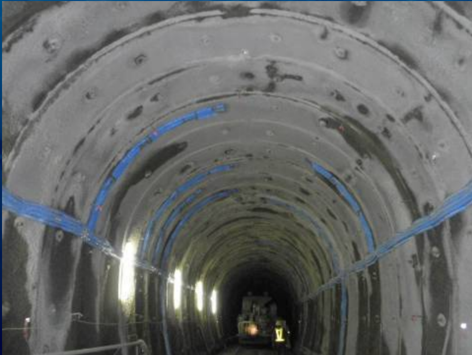
Before Steelfiber shotcrete
